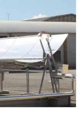
1 m<sup>2</sup> of PTMx can produce over 1000 kWh annually at 150°C, hence avoiding the emission of over 200 kg of CO<sub>2</sub> into the atmosphere<sup>1</sup>.
